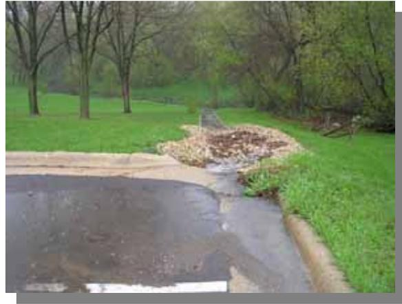
Further study revealed that the rip-rap spillway is the opening to a large underground stormwater storage reservoir. The Community Center was renovated a few years ago, and part of that work included enhanced treatment of runoff from the parking lot and rooftop downspouts. The reservoir does such an effective job that there is no particular advantage in creating a rain garden in the area, short of deconstructing the reservoir and replacing it with the rain garden.
